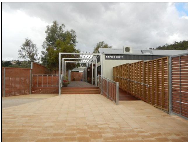
Napier Units at the Thistle Street facility
