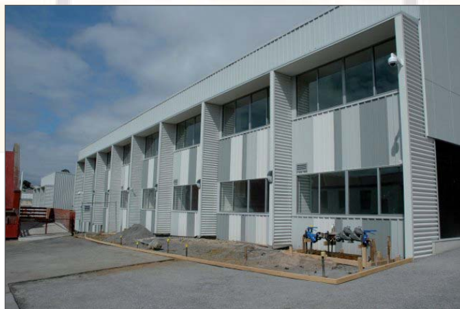
Common Ground Liverpool Street, Hobart.
